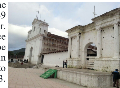
One of the buildings in the Village of Nebaj, Quiche
